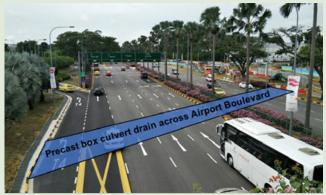
At CAG, besides building the airport on higher platforms above the mean sea level to guard against effects of climate change, the other precaution that we take is to increase the capacity of the airport's drains, to reduce the risk of flooding during intense rain. This is to ensure that Changi Airport continues to operate uninterrupted to serve passengers and customers.
