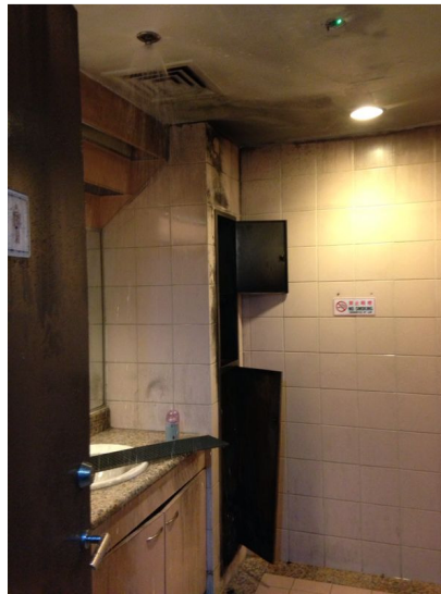
Figure 2 – Heated Smoke from the dustbin fire activated the fire sprinkler and resulted in smoke damage to the property
