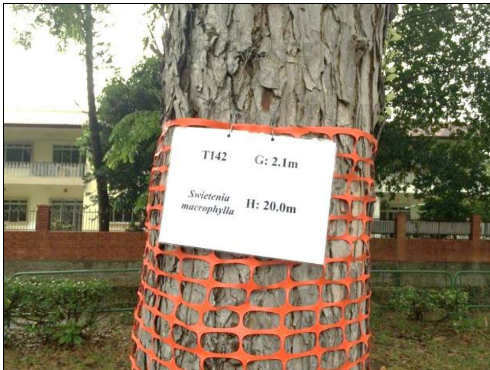
Example of TPZ Preparation
