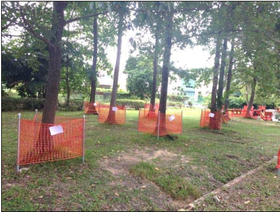
Example of TPZ Preparation
