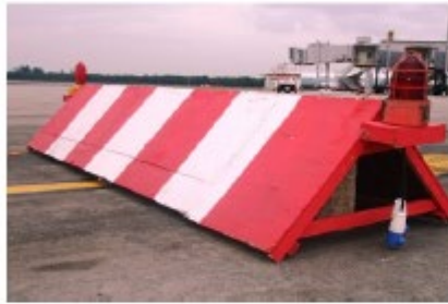
1) Marker board with obstruction lights
