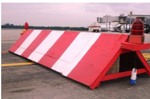
1) Marker board with obstruction lights
