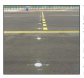
The intermediate holdina position is a dashed white or yellow line marked across the taxiwav. located near taxiwav intersections. It is a designated position intended for traffic control at which taxiing aircraft and vehicles shall stop and hold until further cleared to proceed by
