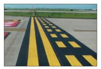
Runway holding position markings contain two solid and two dashed yellow lines across the width of the taxiway. The solid side is closer to the taxiway, while the dashed side is closer to the runway.
