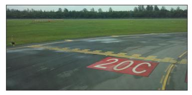
Runway holding positions are designated positions where vehicles must hold and seek clearance from ATC before proceeding into the runway. They are located at all taxiways connected to runways. This is a protective measure to guard against runway incursions. A runway incursion is defined as the incorrect presence of an aircraft, vehicle or person on the runway.
